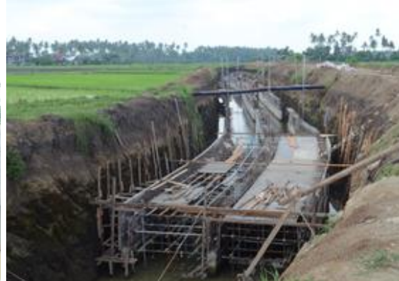
Ongoing construction of the main canal 20.23% completed
