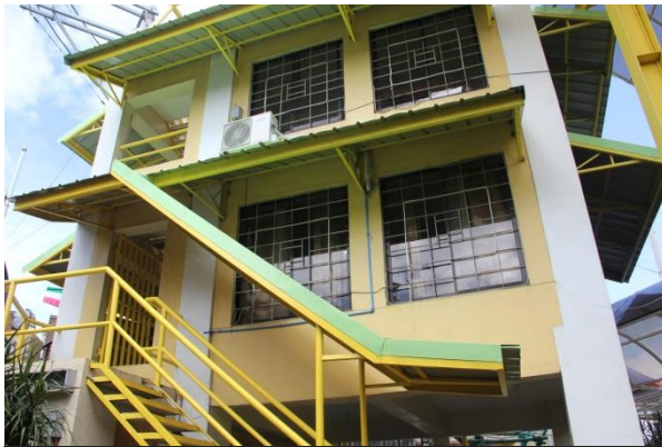
3-storey main building
