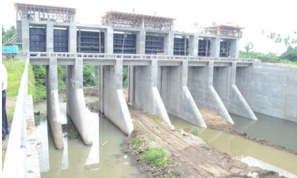
Ongoing construction of the diversion dam 65.37% completed
