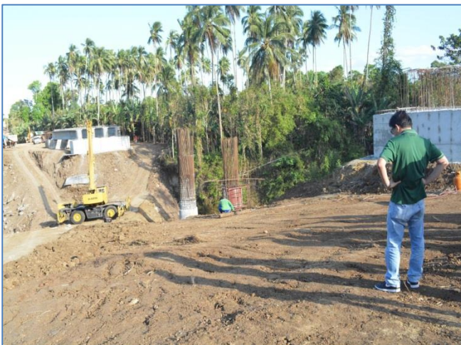
Ongoing construction of the Alaminos-San Pablo Bypass Road
