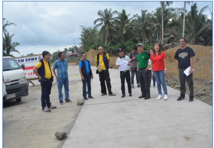
The Calabarzon RPMC inspecting the Lopez Bypass Road
