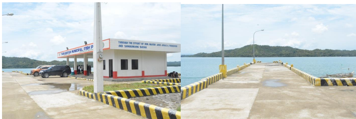
Main building and pier of the Tagkawayan Municipal Fish Port
